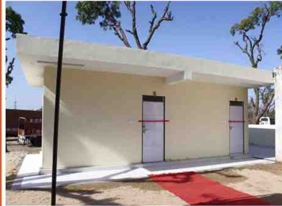
Toilet Block at Bagru Police Station, Jaipur
